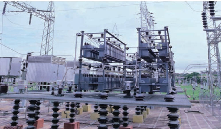
Fixed Series Compensation Scheme at Ballabgarh
